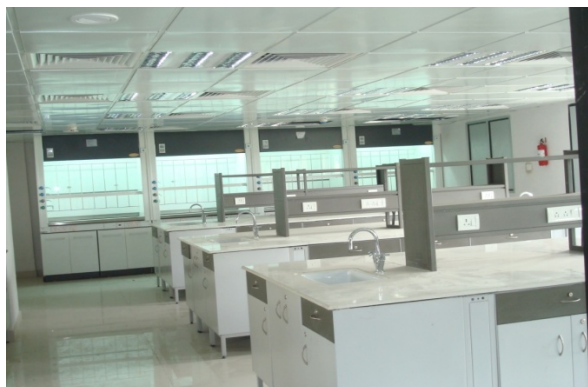
Epoxy coated ,acid & alkali proof, laboratory Tables
