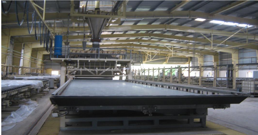
Figure 12: Plant and machinery used for plaster board/ panel manufacturing using phosphogypsum
