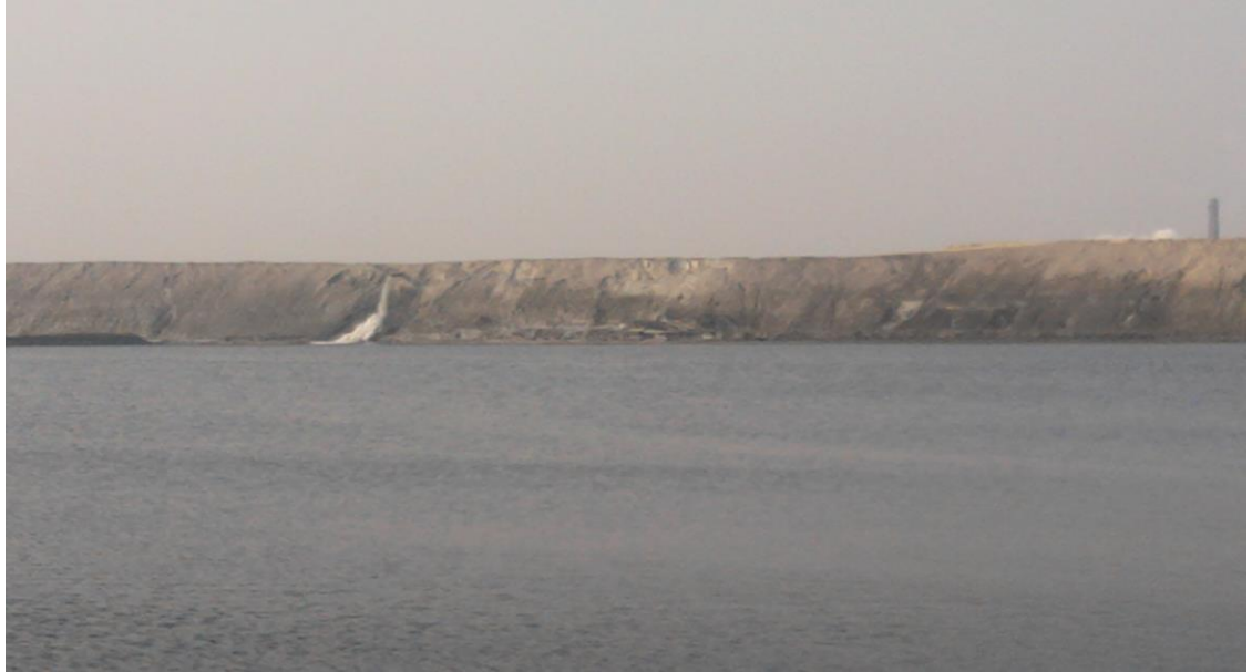
Figure 10: Decanted water collection in 'surge pond' over the phosphogypsum stack
