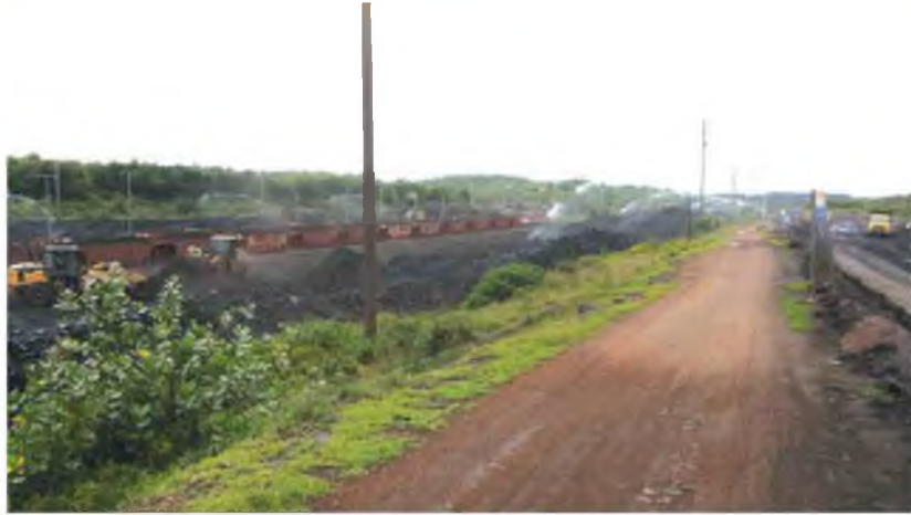
Fig-5.11 Rake loading facility in Railway siding in Bharatpur OCP
