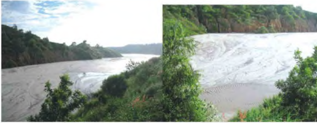
Fig-5.8 Ash filling in abandoned South Balanda Coal Mine Voids in Talcher area
