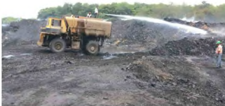
Fig-5.12 Fire fighting at coal stockyard through deployment of fire tender
