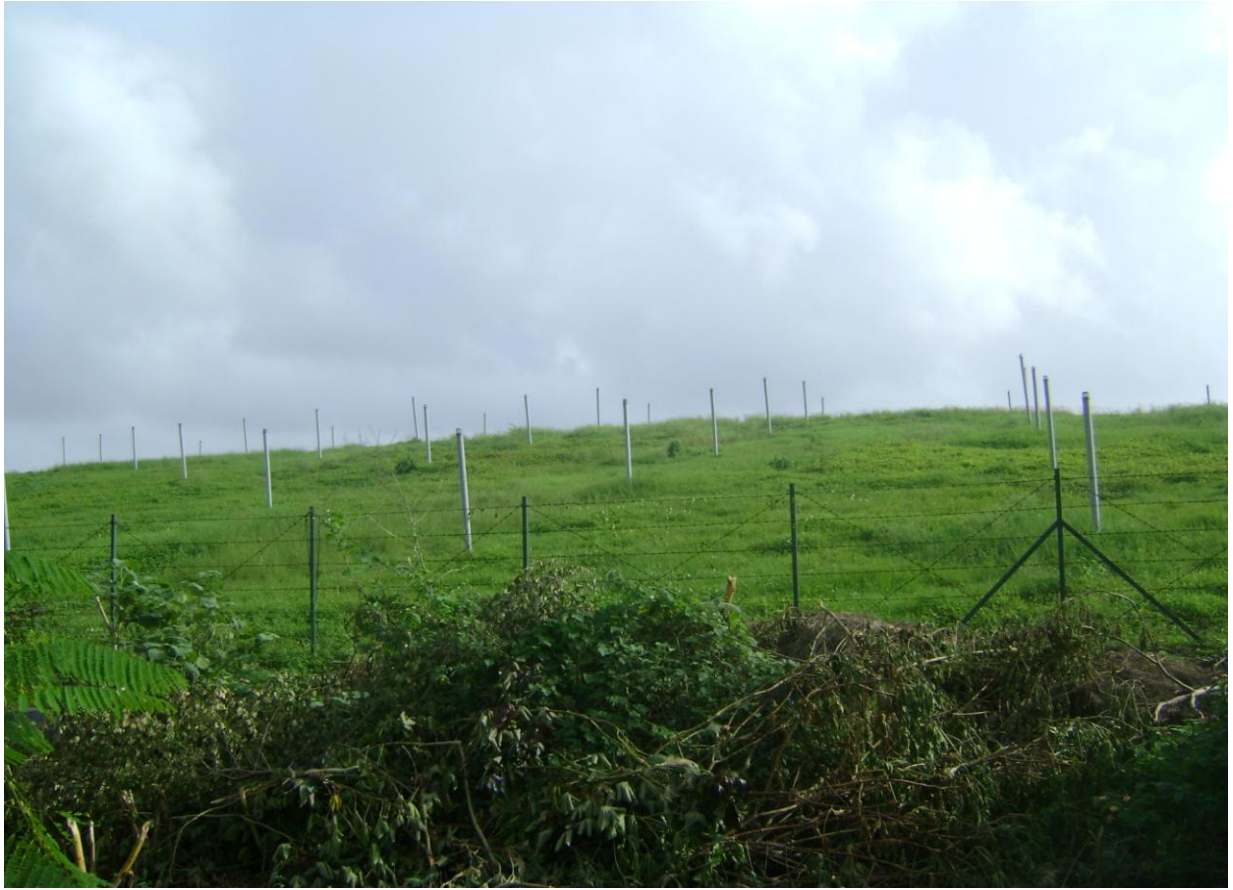
Secured landfill site after encapsulation
