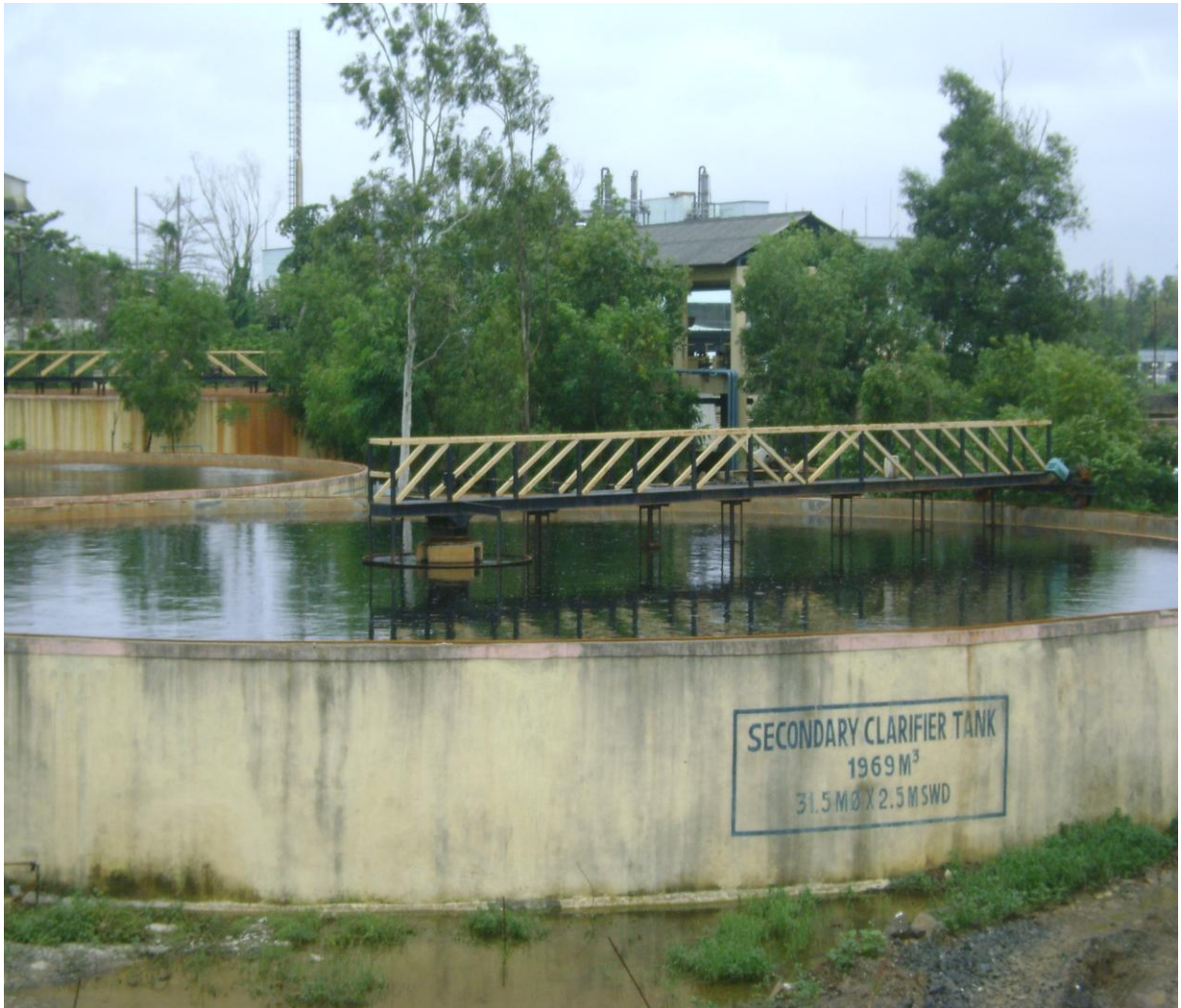
Aerial View of secondary clarifier Tank
