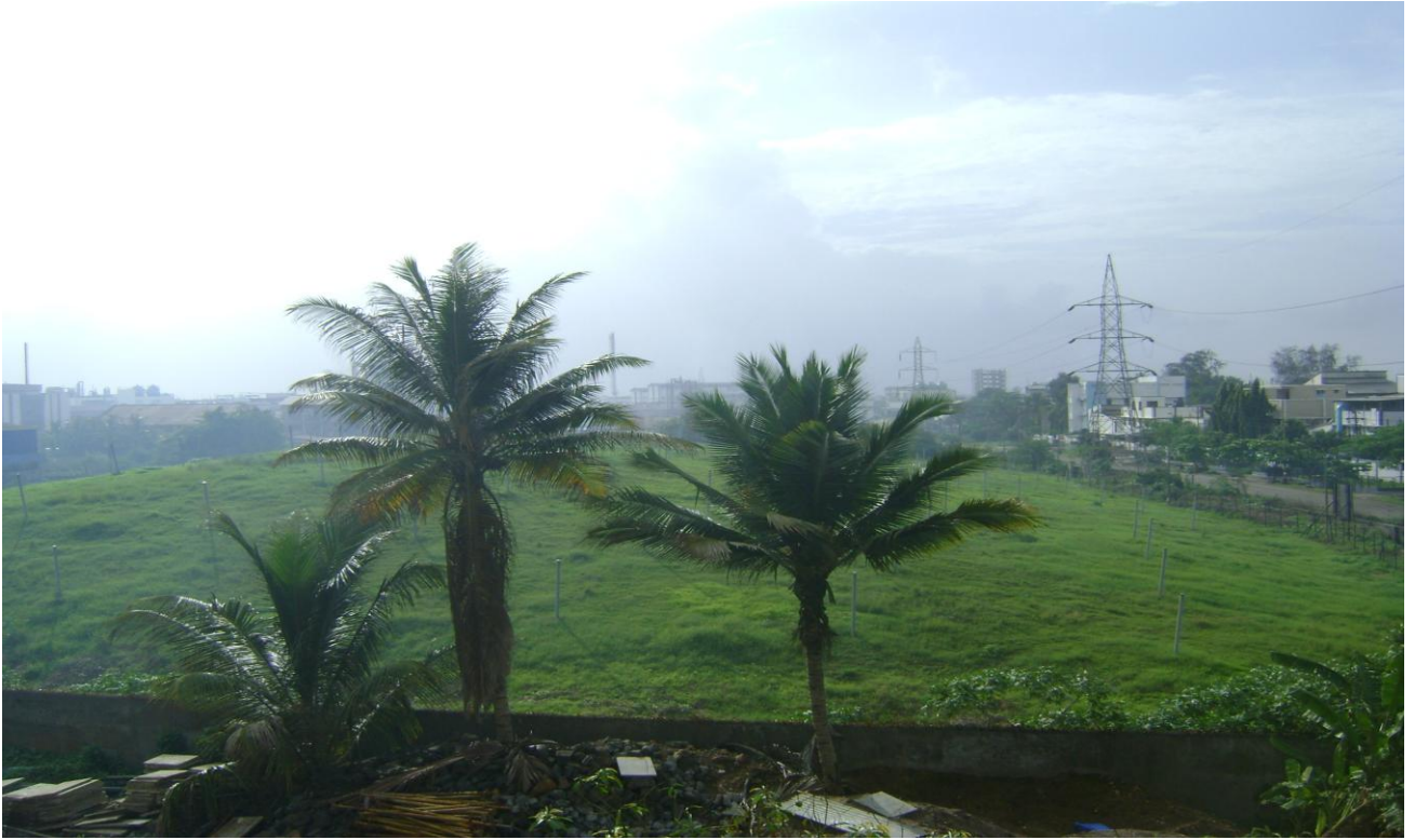
Secured landfill site after encapsulation
