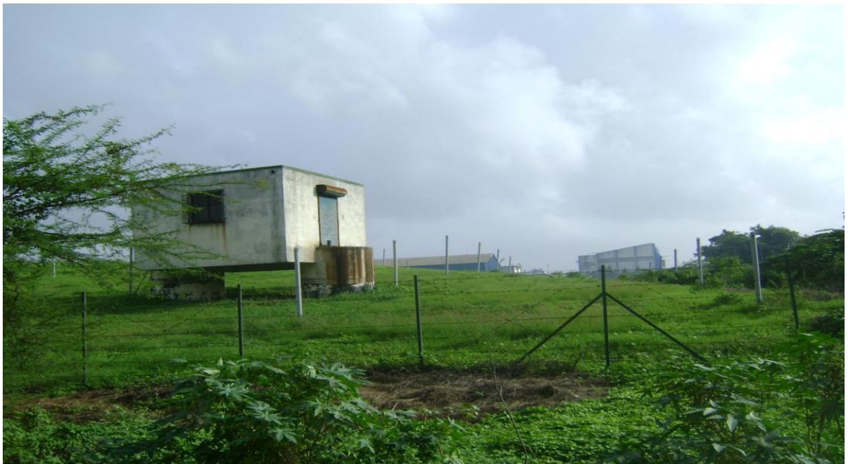
Secured landfill site after encapsulation
