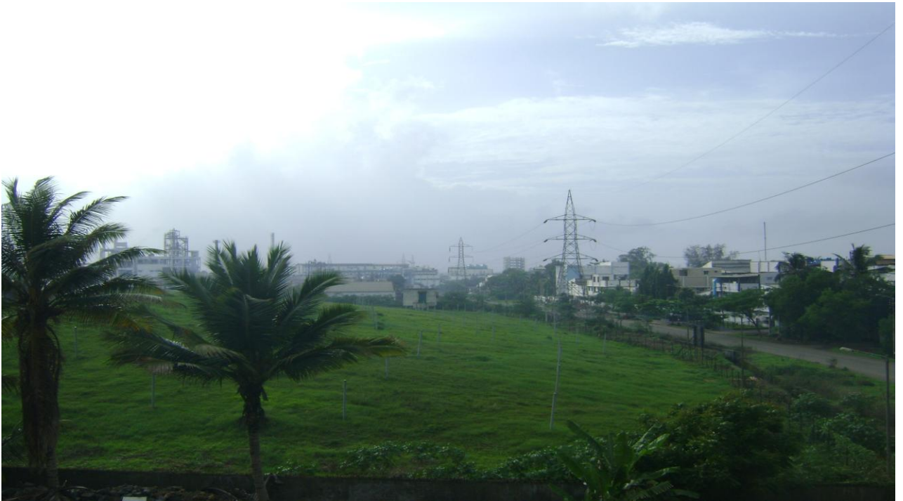
Secured landfill site after encapsulation
