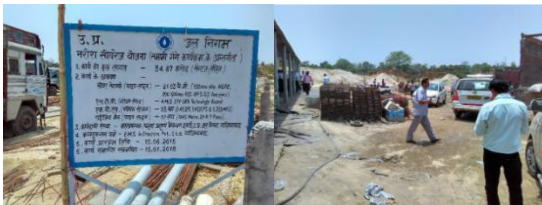
Under construction STP at Narora
