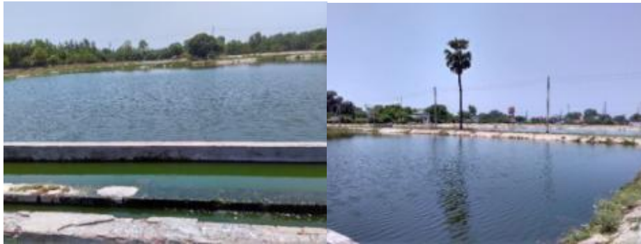
Oxidation ponds at STP-II in Zone-B of Anupshahar
