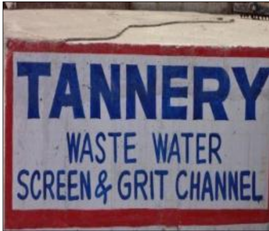
Grit Chamber of CETP Jajmau
