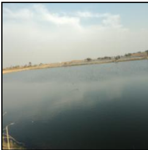
Photograph-View of oxidation pond
