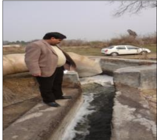
Outlet of CETP
