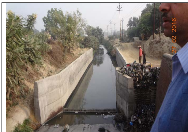
Photo 7: Conveyance system for Bingawa STP
