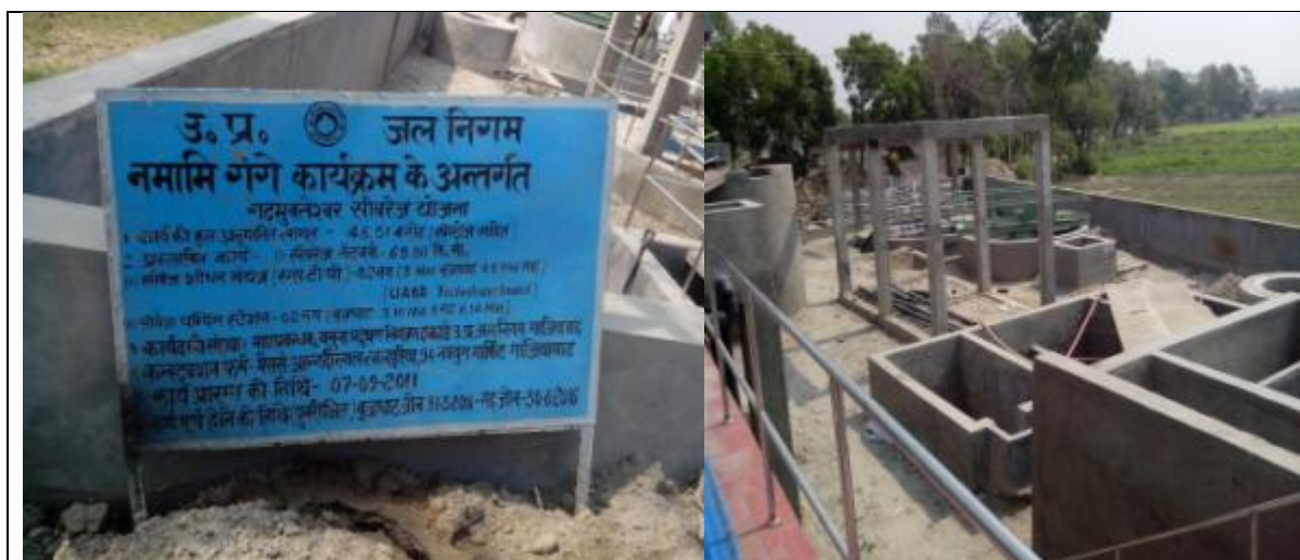
Under construction STP of 3.14 MLD at Brijghat
