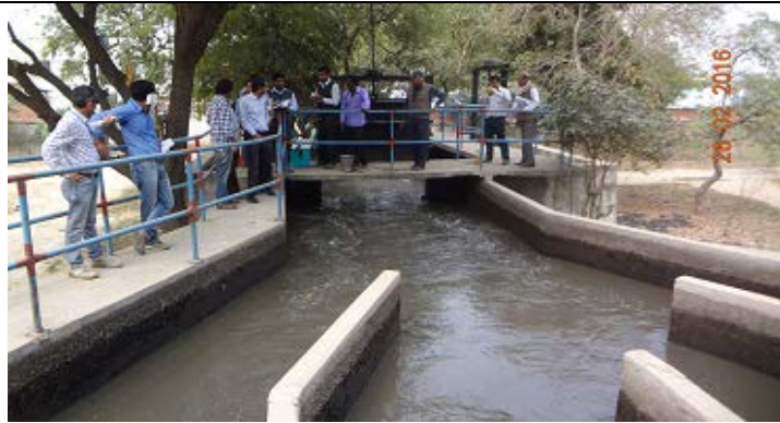
Inlet of STP
