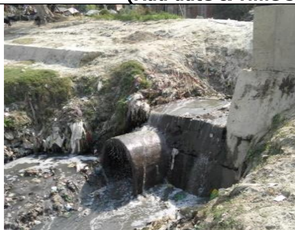
Fig- Sampling point of Gola Ghat Drain
