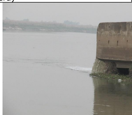
Sisamau drain at Confluence point
