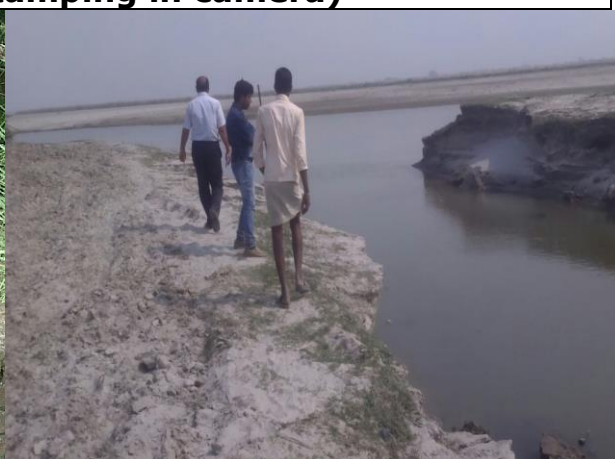
Confluence point of hathikhana drain at Gariyakhare vill
