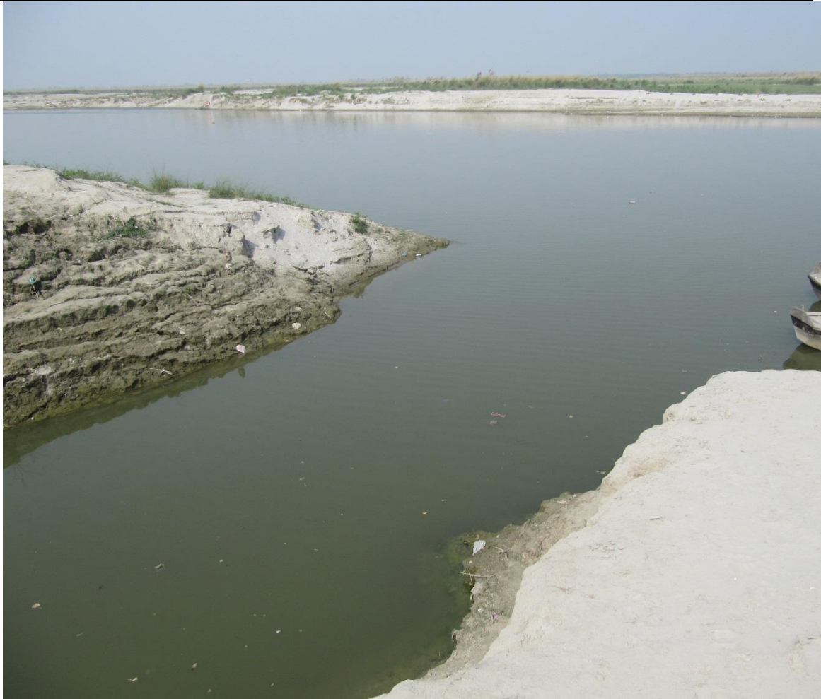
River water backflow into Dabka Drain at Confluence point
