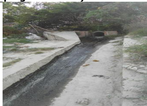
Fig-Confluence point of Jail Drain & River Ganga
