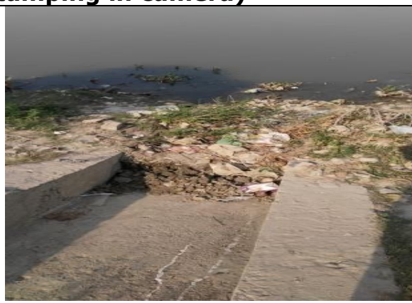
Fig- Confluent point of Police Drain & River Ganga.
