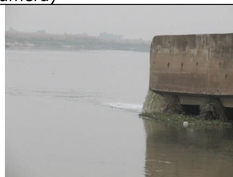
Sisamau drain at Confluence point
