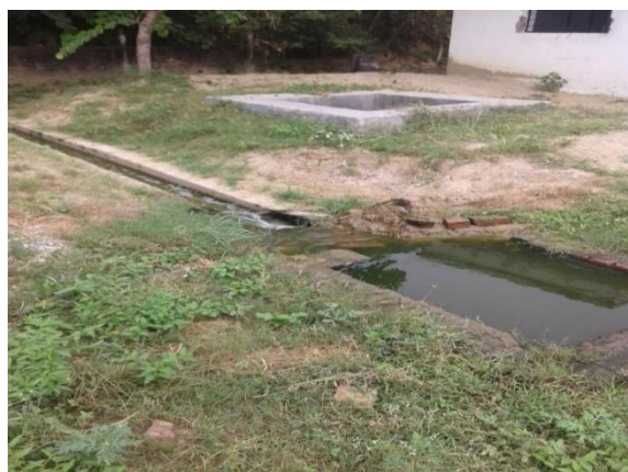
Outlet of STP Drain 1 (Chamunda) (No confluence)
