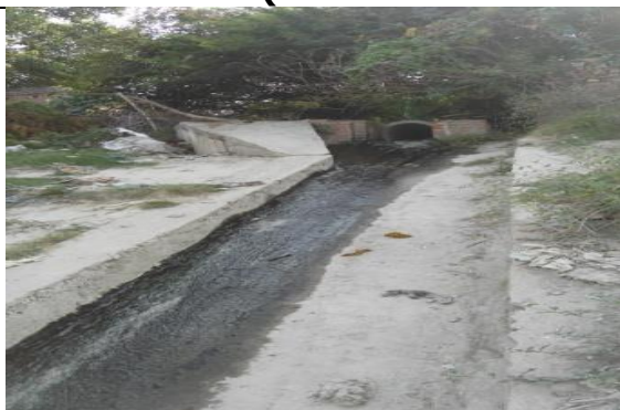
Fig- Sampling point of Jail Drain
