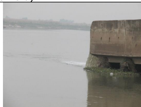
Sisamau drain at Confluence point
