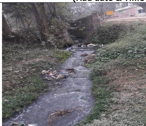
Vivekanand Hospital drain (Right) 100 metres before confluence
