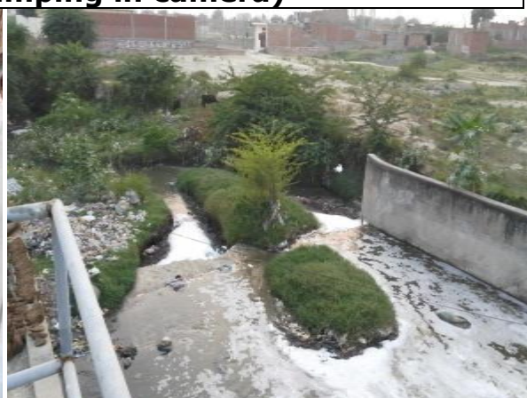
Fig- Near Confluence point of Halwa Khanda Drain & R. Pandu
