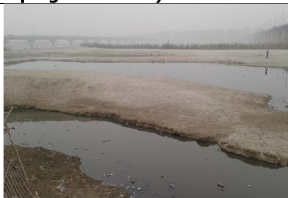
Pic.: The wastewater was storage of Railway Bridge drain in a pond like structure, approximately 150-200 meters away from the left bank of R. Ganga
