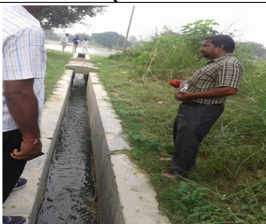
Outlet STP Drain – 2 (Sohan Tau ka Matth) Confluence with Ganga
