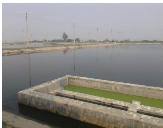
STP Drain – 2 (Sohan Tau ka Matth)
