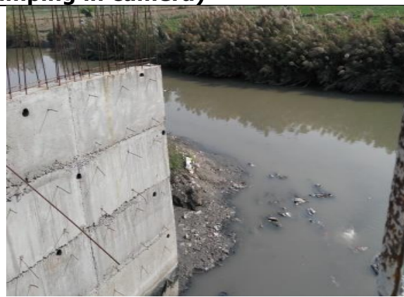
Fig- Confluence point of Panki Drain with River Pandu
