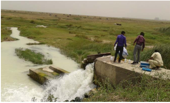
NTPC Shaktinagar Ash Dyke Overflow (SW-9)
