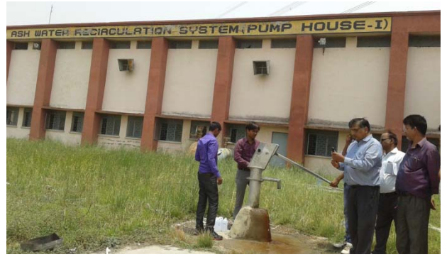
Handpump, NTPC Vinghyanagar ARS (GW-14)
