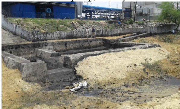
Moher & Moher Coal Settling Pit
