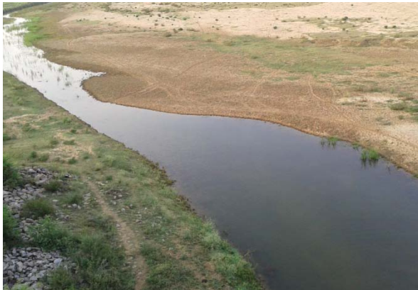
Channel under Rihand River Bridge (SW-19)
