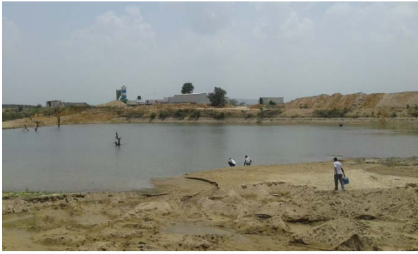
Moher & Moher Sedimentation Tank
