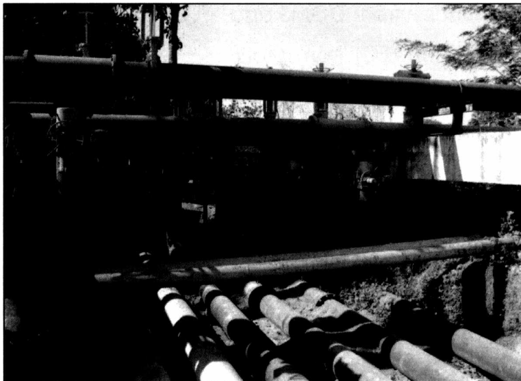
Pumping Station inside NALCO, CPP for Mine Void Filling
