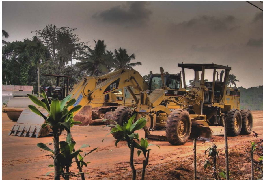
Vallarpadam container transshipment terminal 4 lane road construction at Manjummel, Eloor
