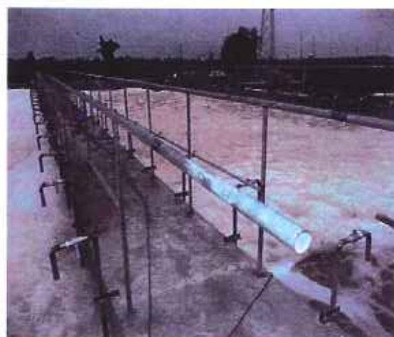
NITRIFICATION /DENITRIFICATION AERATION TANK To reduce TKN & Ammoniacal nitrogen
