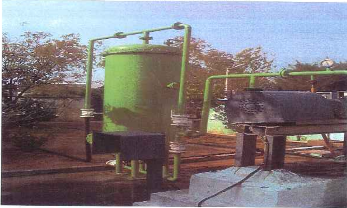
SAND FILTER – To Remove TSS
