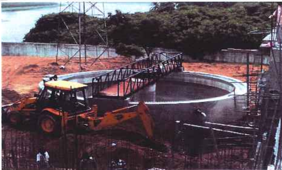
CLARIFIER (Previous Stage ) To reduce TSS
