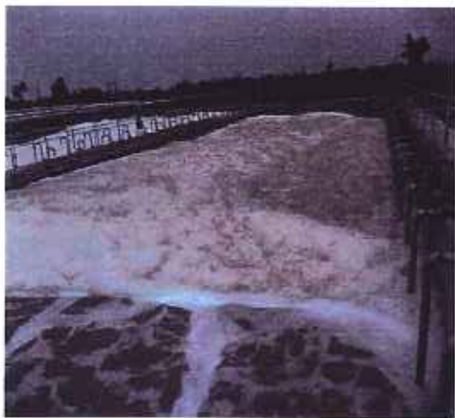
NITRIFICATION /DENITRIFICATION AERATION TANK To reduce TKN & Ammoniacal nitrogen
