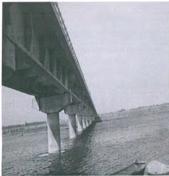
Fig 1- Bithoor Ghat Bridge at Length
