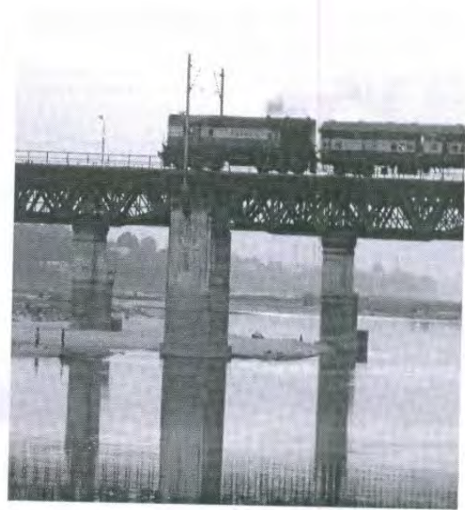
Fig 2- Railway Bridge at Shuklagani
