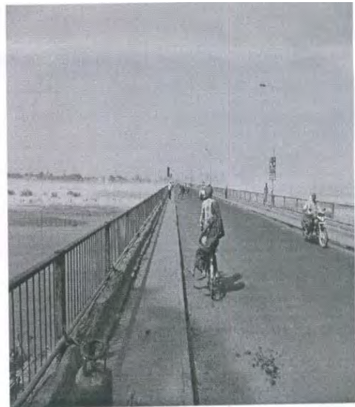
Fig 2- Ghatiya Ghat bridge
