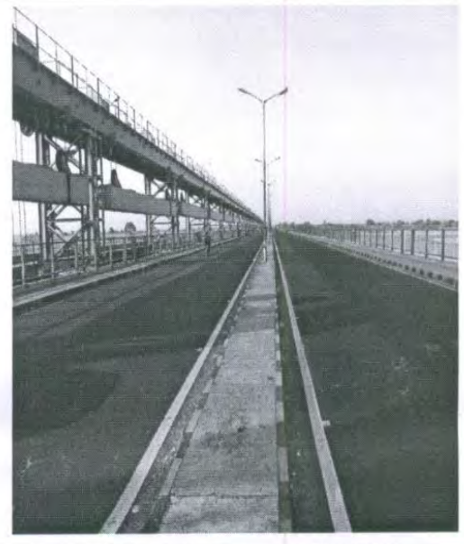
Fig 2- Ganga Barrage Bridge at Top
