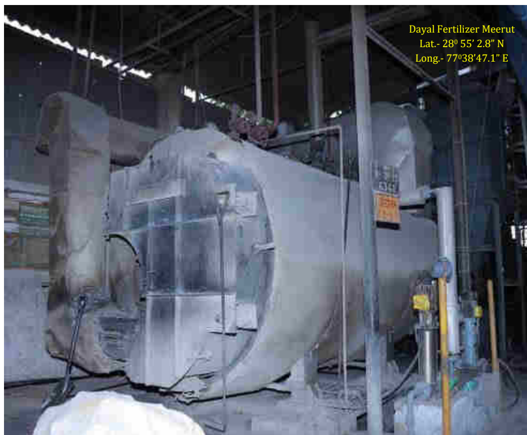
Figure 22: Boiler of M/s Dayal Fertilizers (Capacity 1.5 TPH) in Meerut city
