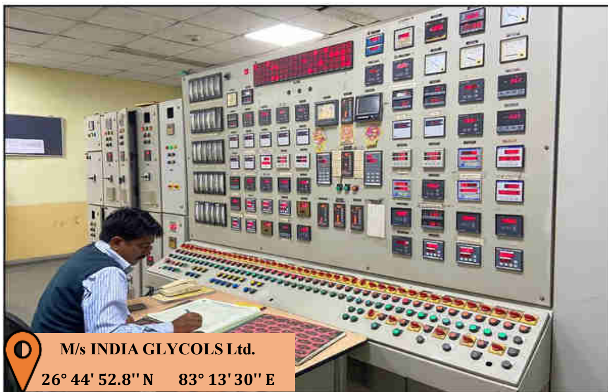
Figure 18: Electrostatic precipitator (ESP-APCS) control panel in M/s India Glycols Ltd., E-1, Sector-13, GIDA, Gorakhpur
