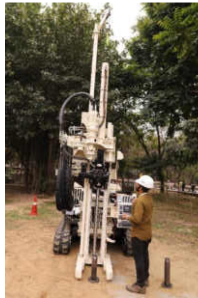
(f) Pushing Dual Tube into the Sub-surface Soil
