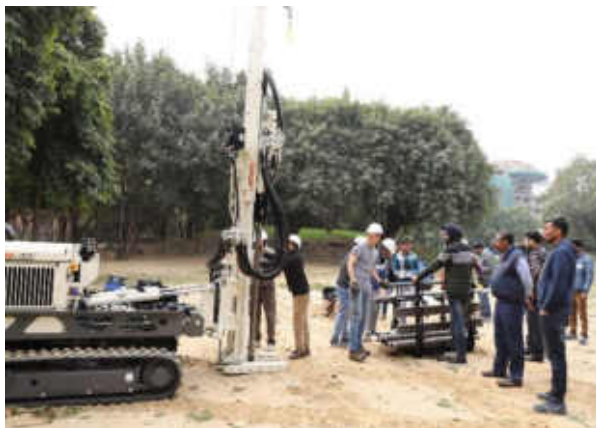
g. Direct push sampling underway
