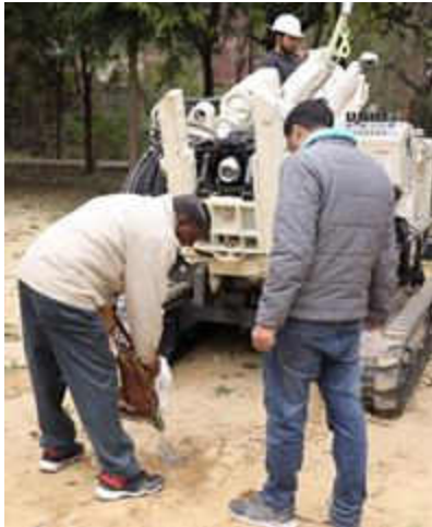
o. Backfilling of borehole
