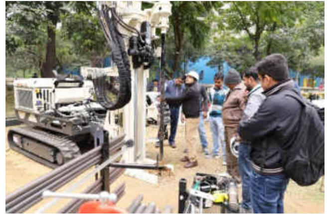
(n) Removing Anchors
