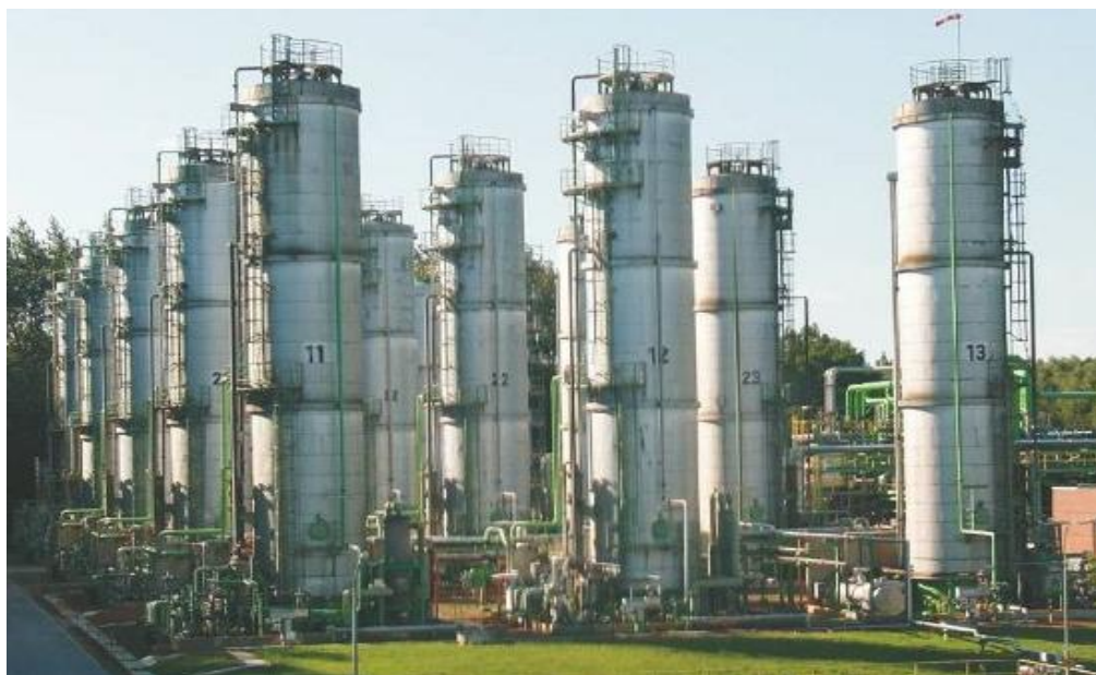
Fig. Representative of Oxidation units in which cumene hydroperoxide is produced. Source, http://www.essentialchemicalindustry.org/chemicals/phenol.html .
