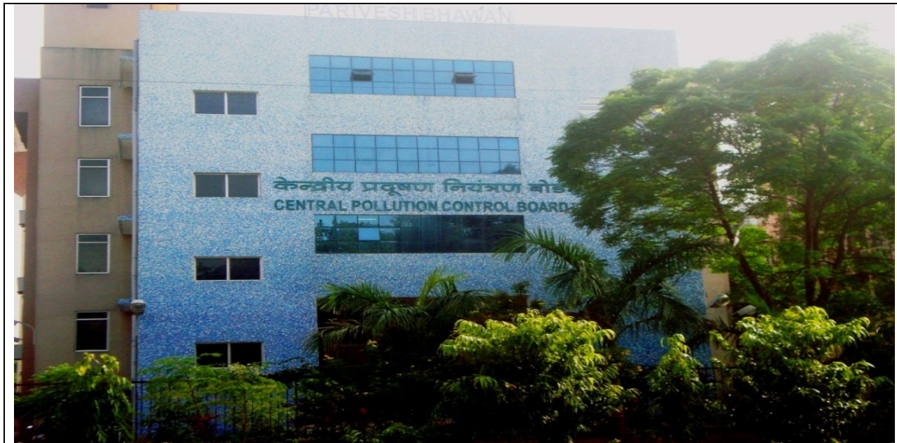
Zonal Office (W) Building at Vadodara
