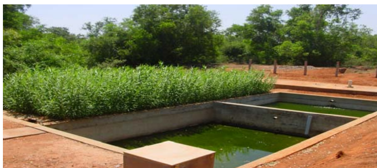
WASTEWATER TREATMENT UNIT
