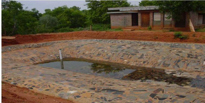
RAINWATER HARVESTING POND
