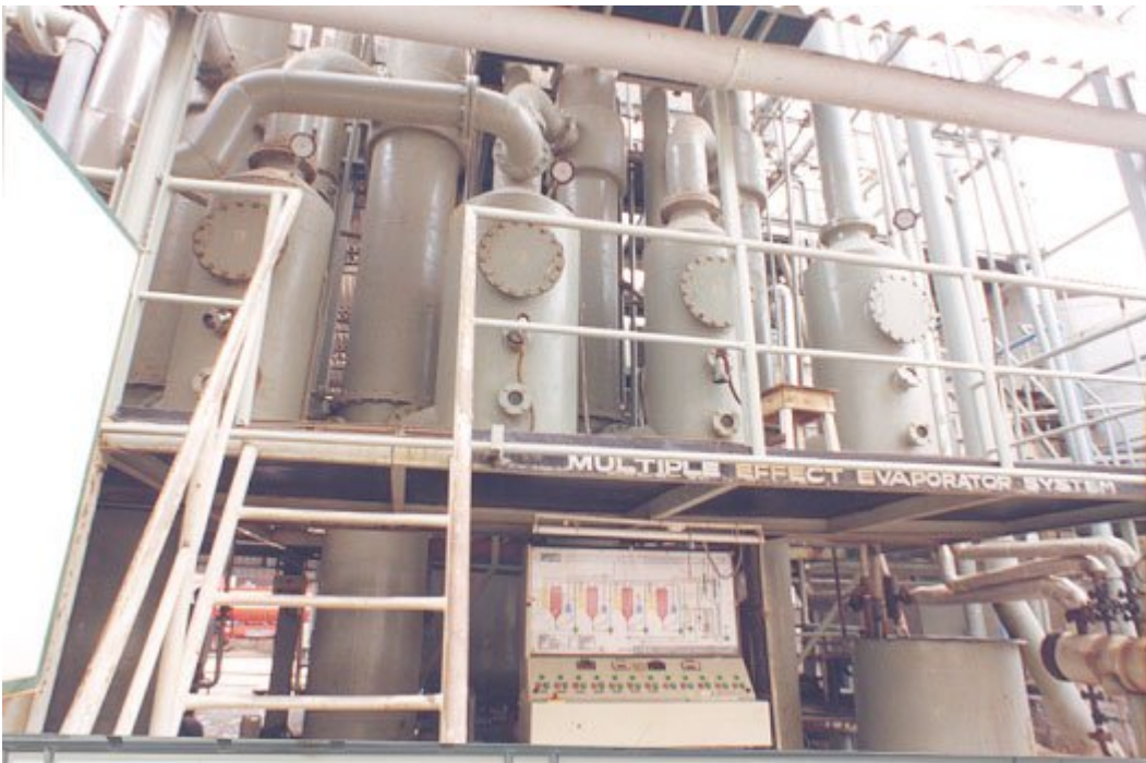
Multiple Effect Evaporator
