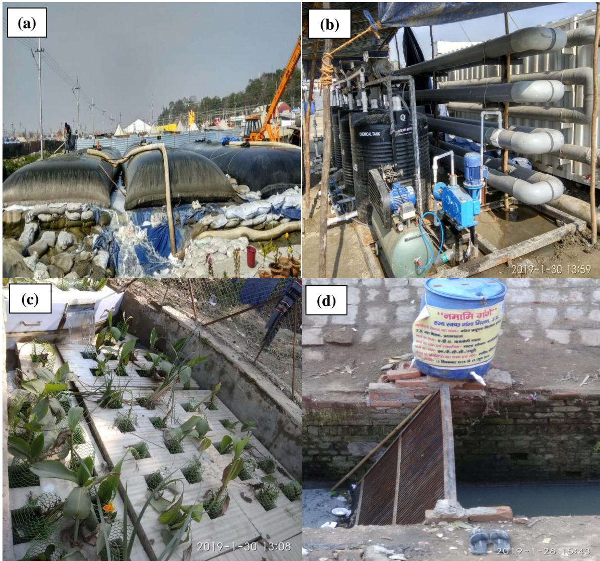
Figure 34 (a & b) Deployment of Geo tubes for treatment of drains directly going towards river; (c) Deployment of phytoremediation for treatment of drains directly going towards river; and (d) Deployment of bioremediation for treatment of drains directly going towards river
