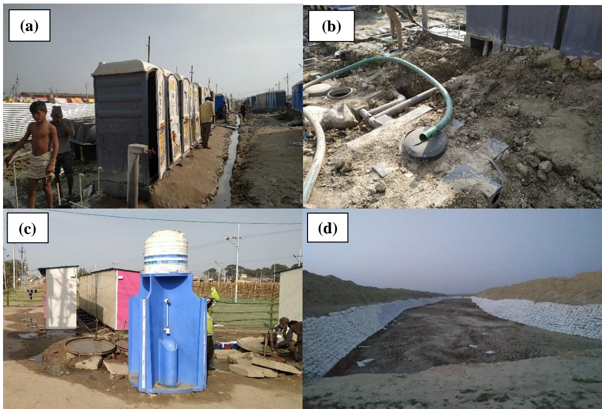
Figure 37 (a) Portable toilets in Kumbh Mela area-2019; (b) Plastic tanks buried in soil connected to portable toilets; (c) Portable urinals in Kumbh Mela area-2019; and (d) Temporary ponds constructed for storage of waste water
