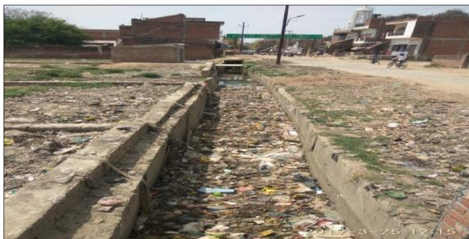
Figure 22 Solid waste dumping in Adanga Nala
