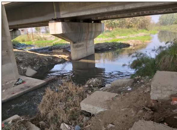
Figure 11 River Kali-East U/s Hapur city Drain
