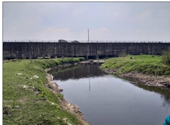
Figure 12 Confluence point of Chhoiya Drain with River Kali-East
