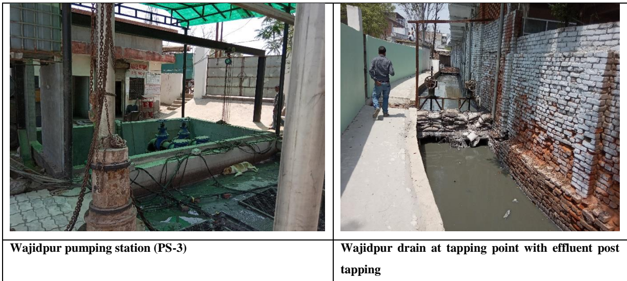
Figure 21 Wajidpur pumping station in Jajmau area, Kanpur
