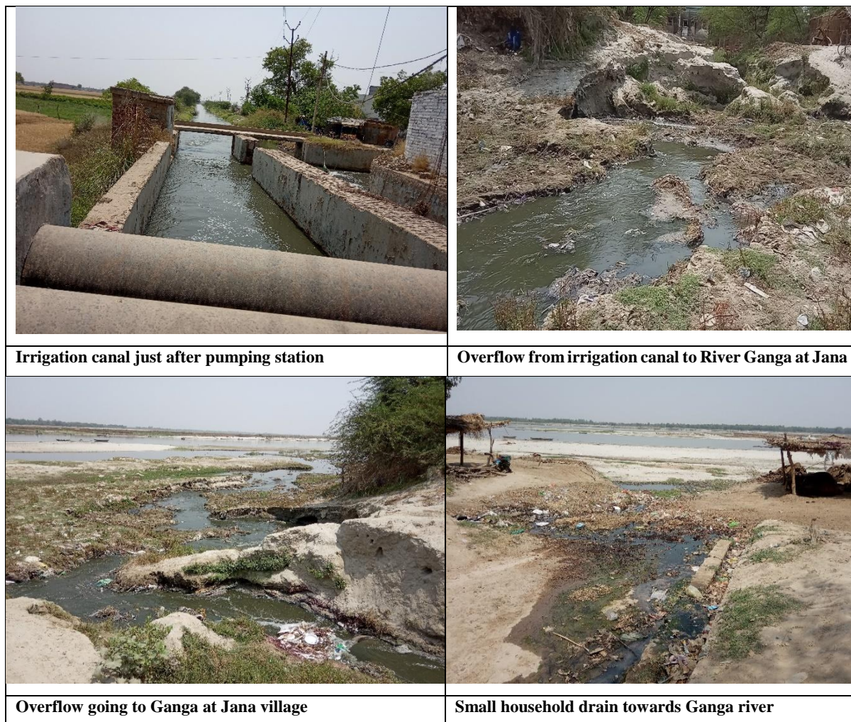
Figure 22 Breach in irrigation channel near Jana village, Kanpur
