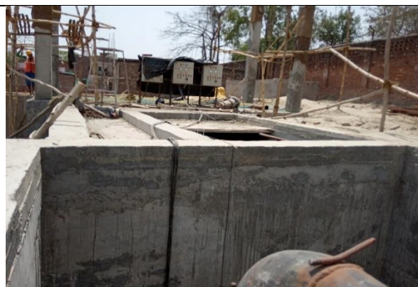
Under construction pumping station at Shitla Bazar Nallah
