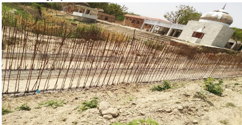
Figure 7 Under construction wetland technology Sewage treatment system on drains at Bithoor
