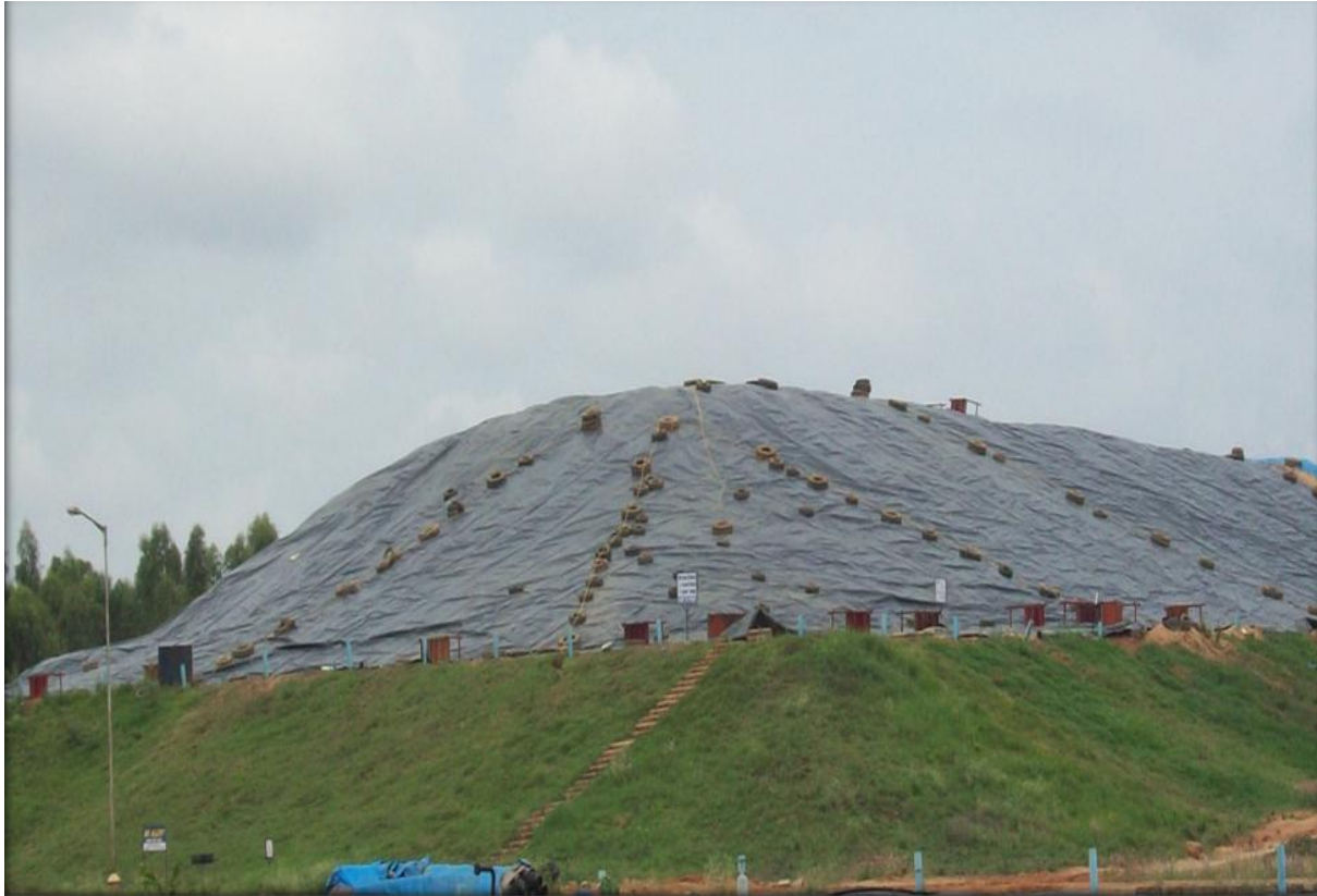
Fig 5: Cells covered with tarpaulins
