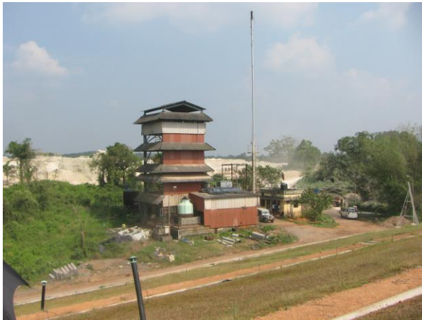
Fig.1: Showing the Leachate treatment system (MEE) with boiler.
