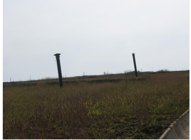
Fig.8: Cells cover is provided gas vents.
