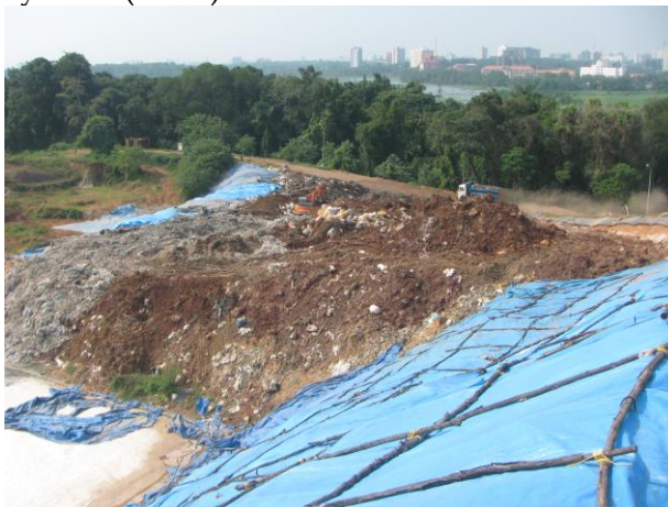
Fig.3: Cell 3 is in operation, temporary cover provided to the cells.
