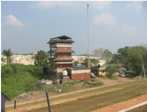
Fig.1: Showing the Leachate treatment system (MEE) with boiler.
