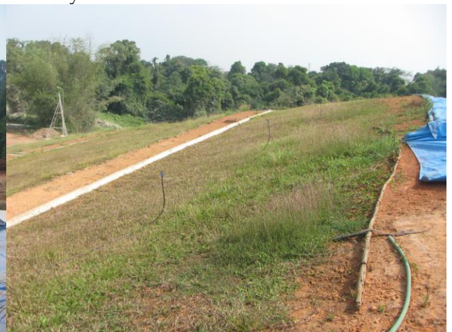
Fig.6: Cells green cover is provided with sprinklers.
