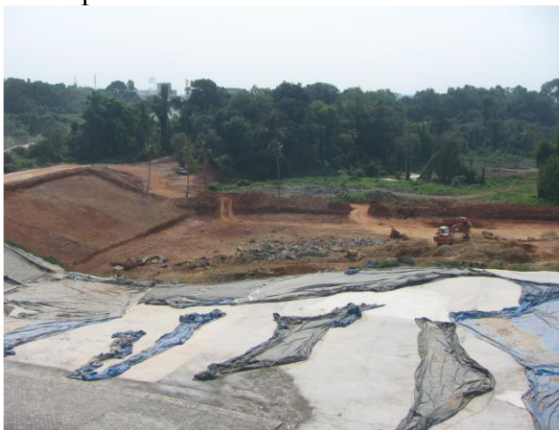
Fig.5: Cells under construction for expansion.
