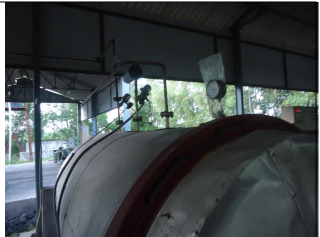
Fig No.3 Pressure guage provided with autoclave
