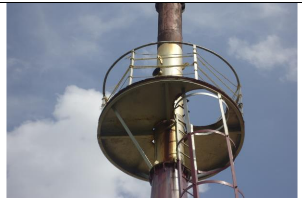
By tying rope around the platform, source emission monitoring carried out
