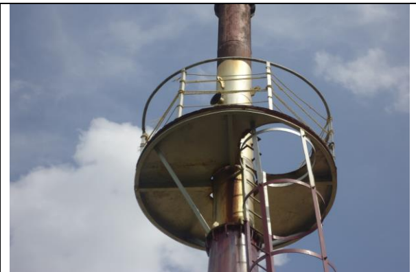
By tying rope around the platform, source emission monitoring carried out
