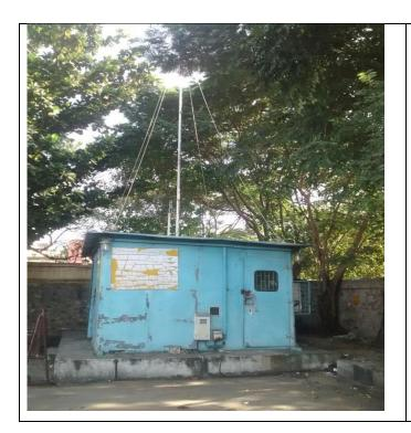
Trees grown up around the monitoring station at Alandur because of which the measurement of met parameters are non-representative. Due to frequent hit by the MTC bus and continuous heavy rain in the area, water leak from roof is observed. The condition of the entire station structure is damaged which require replacement or reconditioning.
