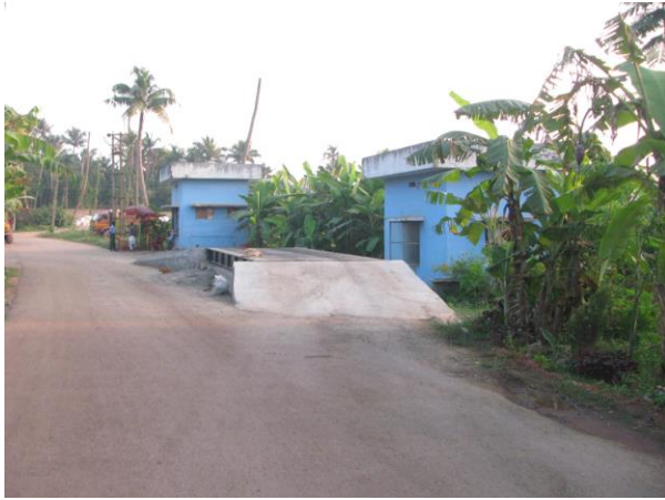
Fig.1 : Weigh Bridge at the entrance
