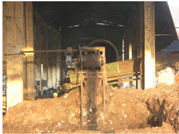
Fig.10 : Compost processing area
