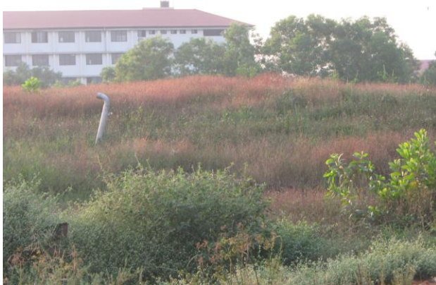
Fig.11 : Old landfill with gas venting system
