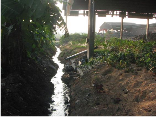
Fig.7 : No proper drain for leachate carrying, Kaccha drain
