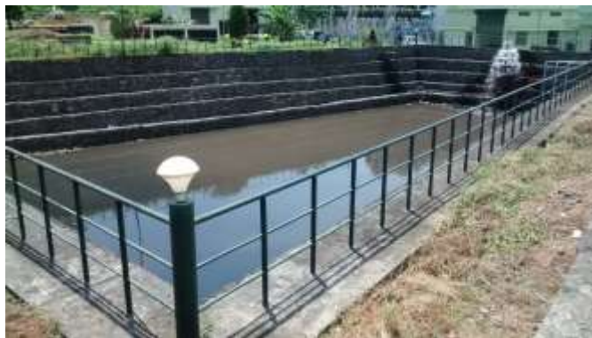
Treated Effluent Recharge Pond
