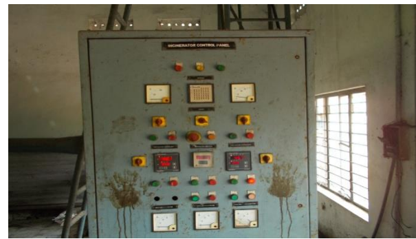
Fig 4: View of Programmable Logic Control
