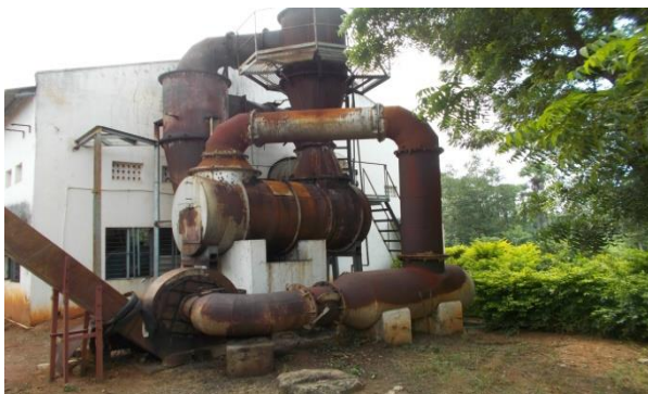
Fig 5: View of APCDs attached with incinerator
