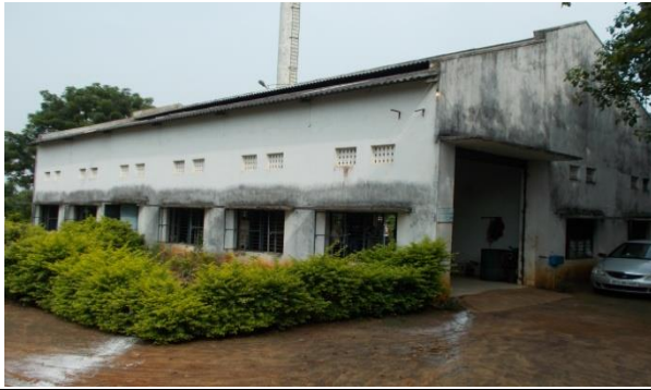
Fig 1: View of the facility
