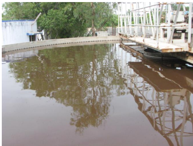
Fig 4: Secondary Clarifier
