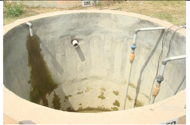
SLUDGE COLLECTION TANK OF PILOT PLANT
