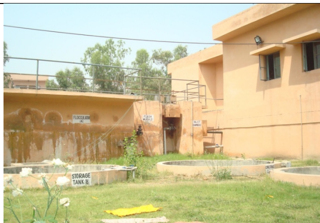
0.5MLD PILOT WATER TREATMENT PLANT BASED ON SRP TECHNOLOGY
