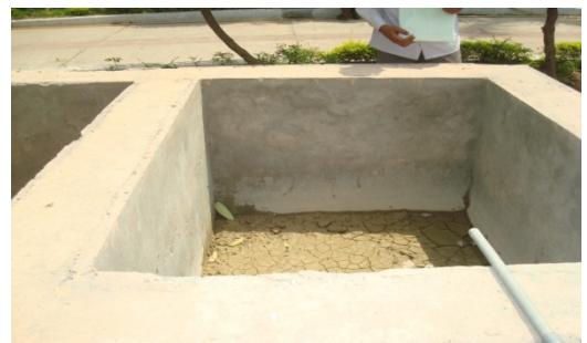
SLUDGE DRYING BED OF PILOT PLANT
