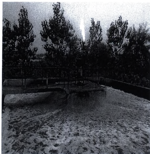
Aeration tank and in the background flaring of Methane Gas
