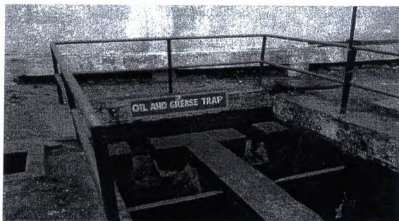
Screen chamber & Oil & Grease trap
