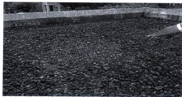
Anaerobic filler tank
