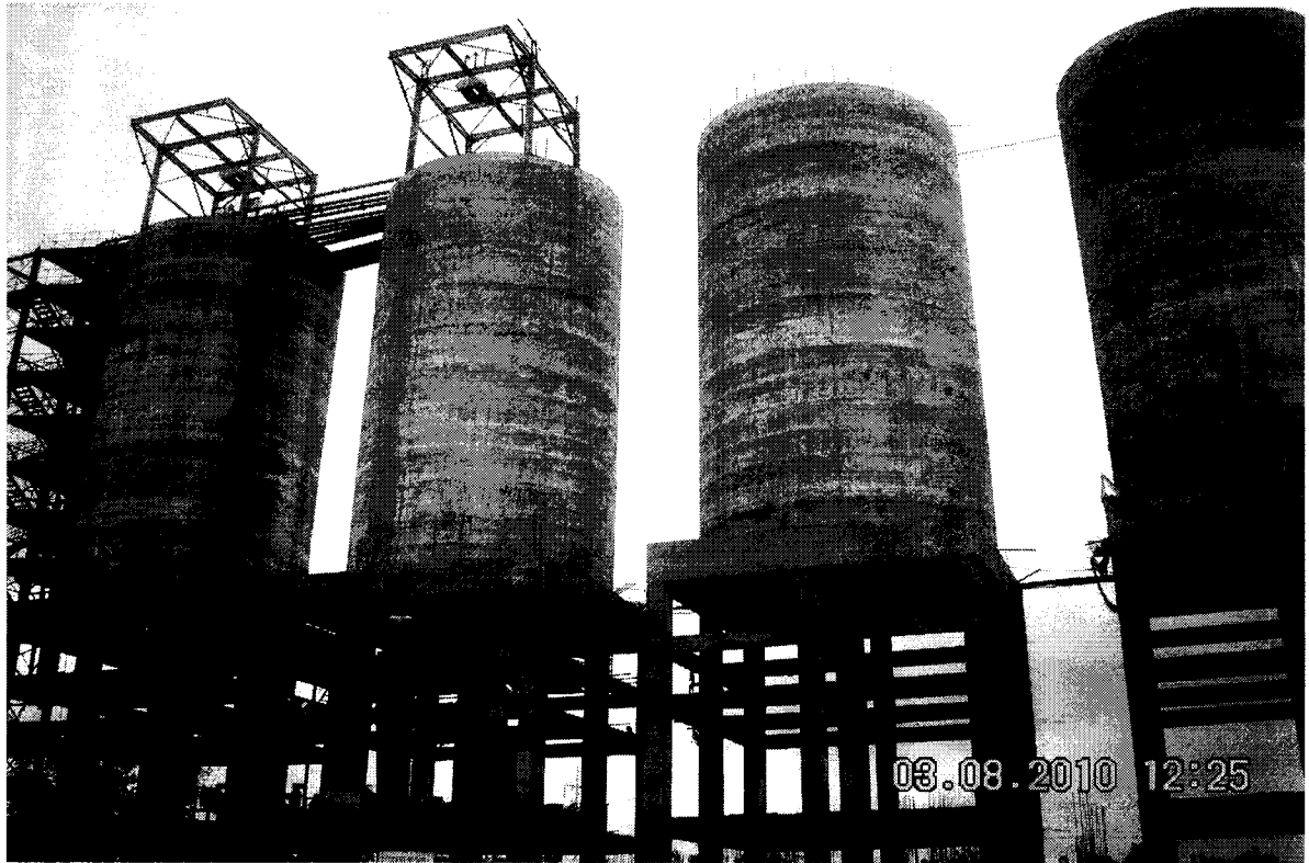
Photo-9 : Construction of silo for dry ash collection of M/s CSEB (W)
