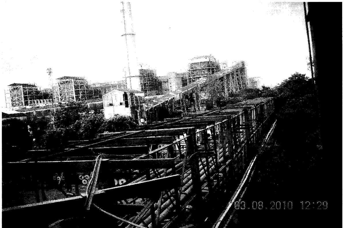
Photo-10 : Construction of conveyer system of M/s CSEB (W)
