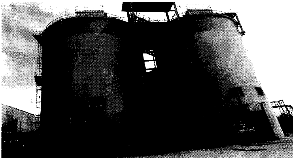
Photo-15 : Ash Silo for collection of dry fly ash of M/s BALCO (540 MW)
