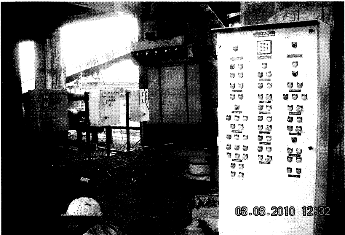
Photo-12 : Installation of control panel for HCDS system of M/s CSEB (W)
