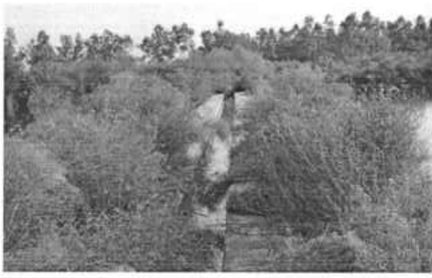
Boundry of Dasuya treatment plant require cleaning
