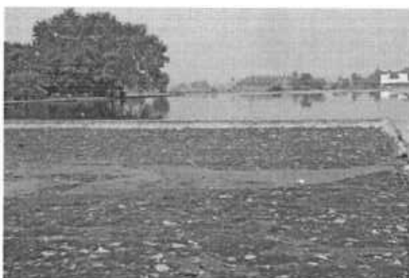
Ponds of Sultanpur Lodhi treatment plant are full of sludge
