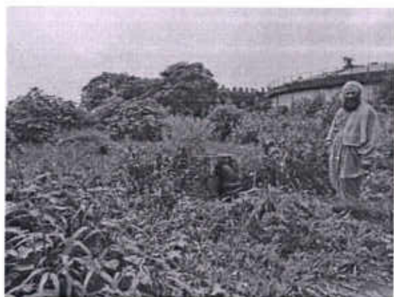
Sludge system of treatment plant of B.B.M.B colony Nangal Roper is not working
