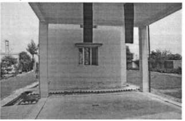
Sludge system of Begowal treatment plant is not working
