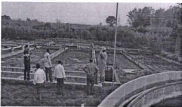
Dried up sludge beds at Maujewal Nangal Treatment Plant
