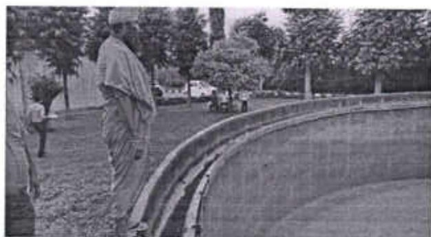
Treatment Plant of Maujewal Nangal is not working
