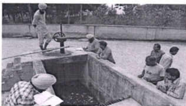
Pumping station of Shamchurasi is not working
