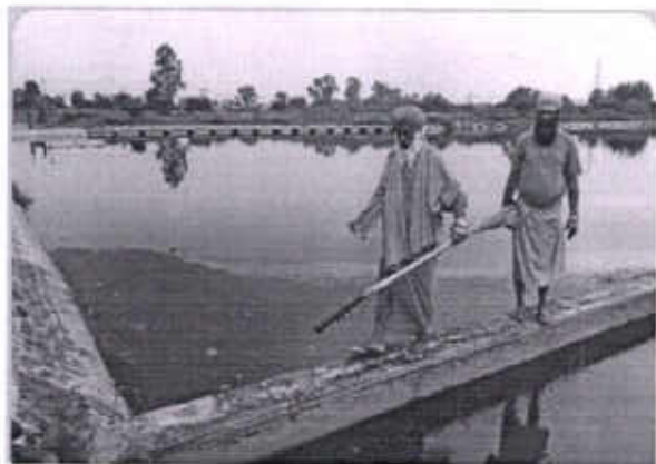
Ponds of 111 M.L.D Pholriwal Treatment Plants Jalandhar are full of Sludge.
