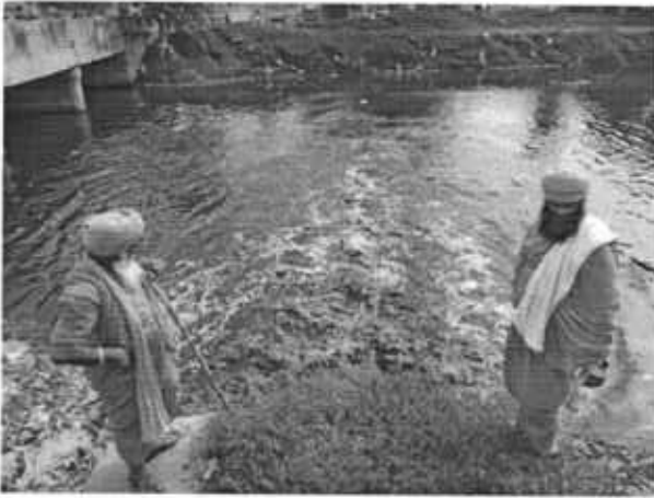
Jamalpur Treatment Plant is out of order, Polluted water is flowing direct into Buddha Nullah Ludhiana
