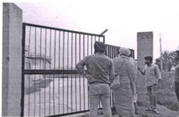
Treatment Plant of Nurmehal Jalandhar is not working and the gate is locked.
