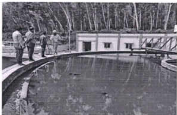
Pond of Brari Nangal STP Roper is full of sludge
