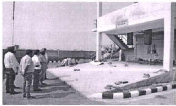
Sludge system of Makhu Treatment Plant is not working
