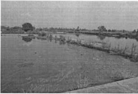
Ponds of Dasuya treatment Plant are full of sludge
