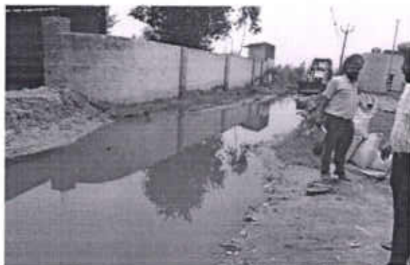
S.T.P of Phillaur Jalandhar (South Area) being not in operation ,dirty
