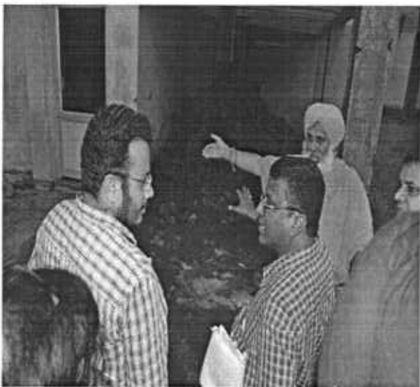
Sludge System of STP 50 MLD of Basti pir daad Jalandhar is not working regularly.
