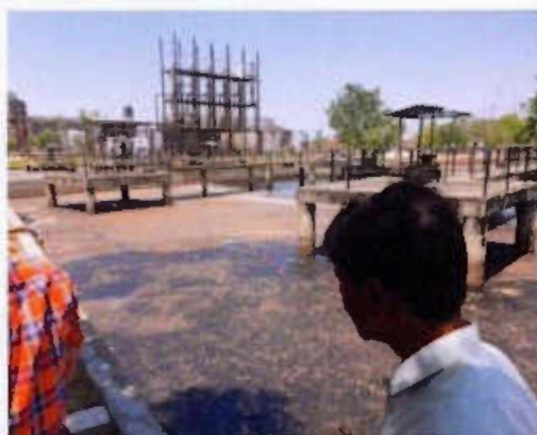
Plate-7: One big tank full of water adjacent to the aeration tank-1
