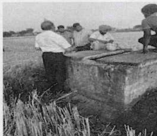
Plate-2: Photograph showing the manhole provided on the drain leading to Saraswati river.
