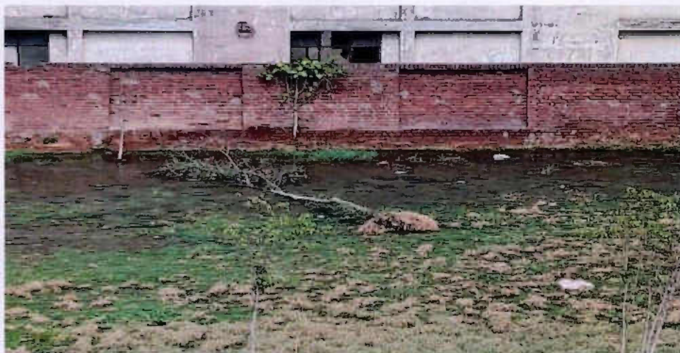
Plate-9: Stagnation of effluent onto Land
