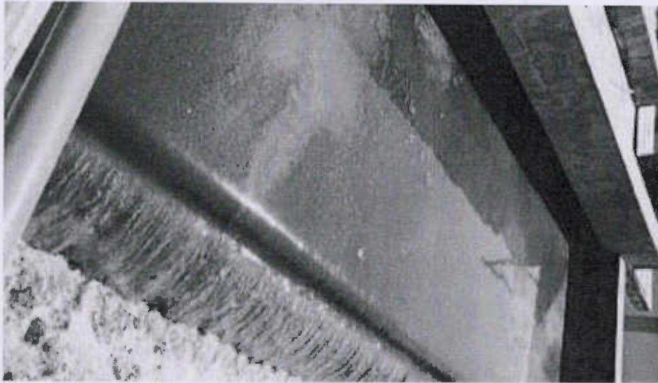
Plate-I: Effluent after screening and grit chamber containing lot of solid particles.
