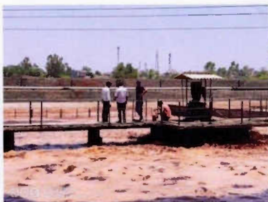
Plate-5: Aeration Tank-1
