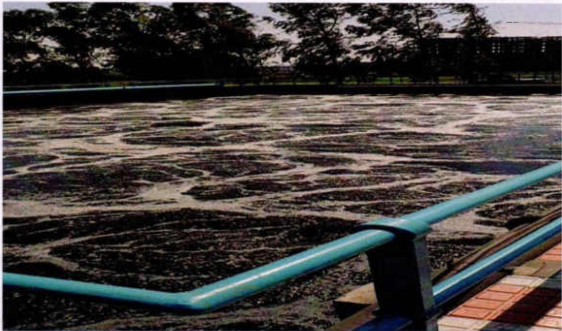
Plate-2: Effluent in aeration chamber black in colour
