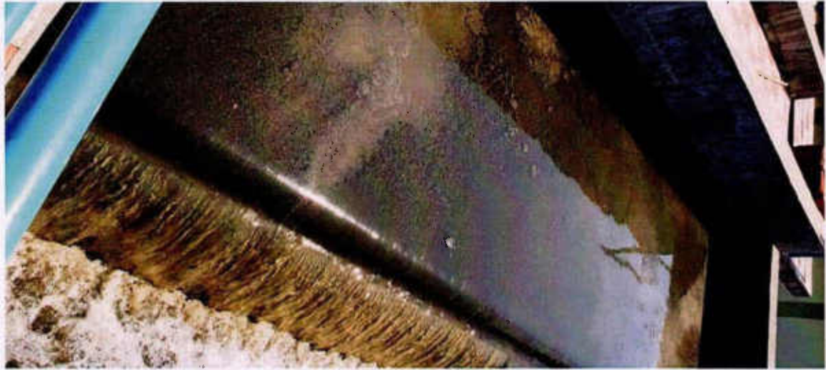
Plate-I: Effluent after screening and grit chamber containing lot of solid particles.
