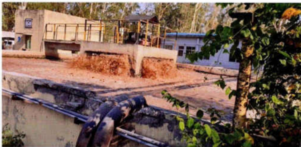
Plate-2 :Aeration Tank
