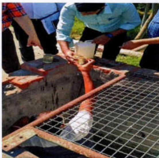
Plate-1: Final outlet of ETP
