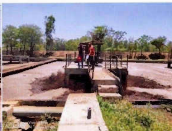
Plate-6: Aeration Tank-2
