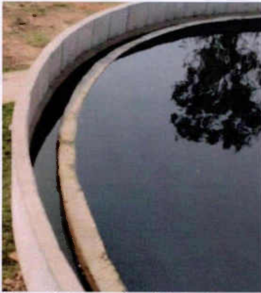
Plate-3: Dry weir of the primary Clarifier
