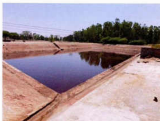
Plate-8: Lagoon for storage of spent wash
