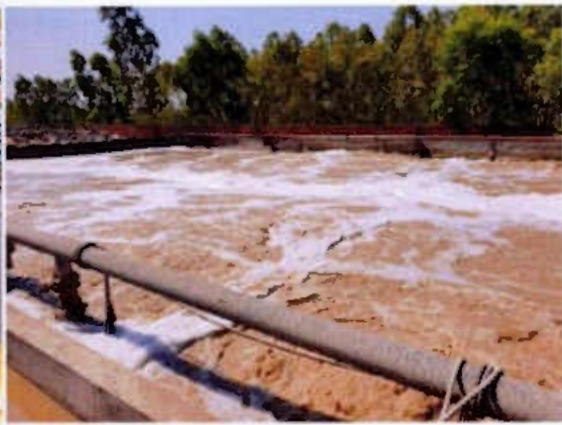
Plate-10: Aeration Tank-1
