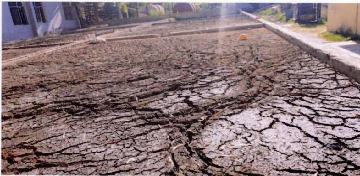
Plate-6 : Sludge Drying Beds full of sludge
