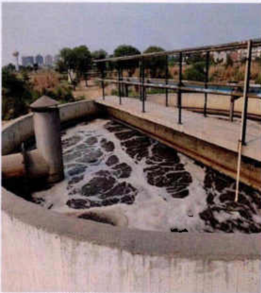
Plate-5: MBBR-2 tank
